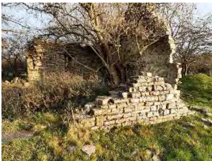
Image 16: Ruined Building, B1
