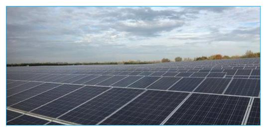
Figure 11 - Typical View of Arrays with Joints which Distribute Runoff
